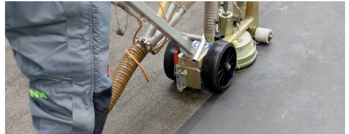
Aquablast - manual surface cleaning equipment
