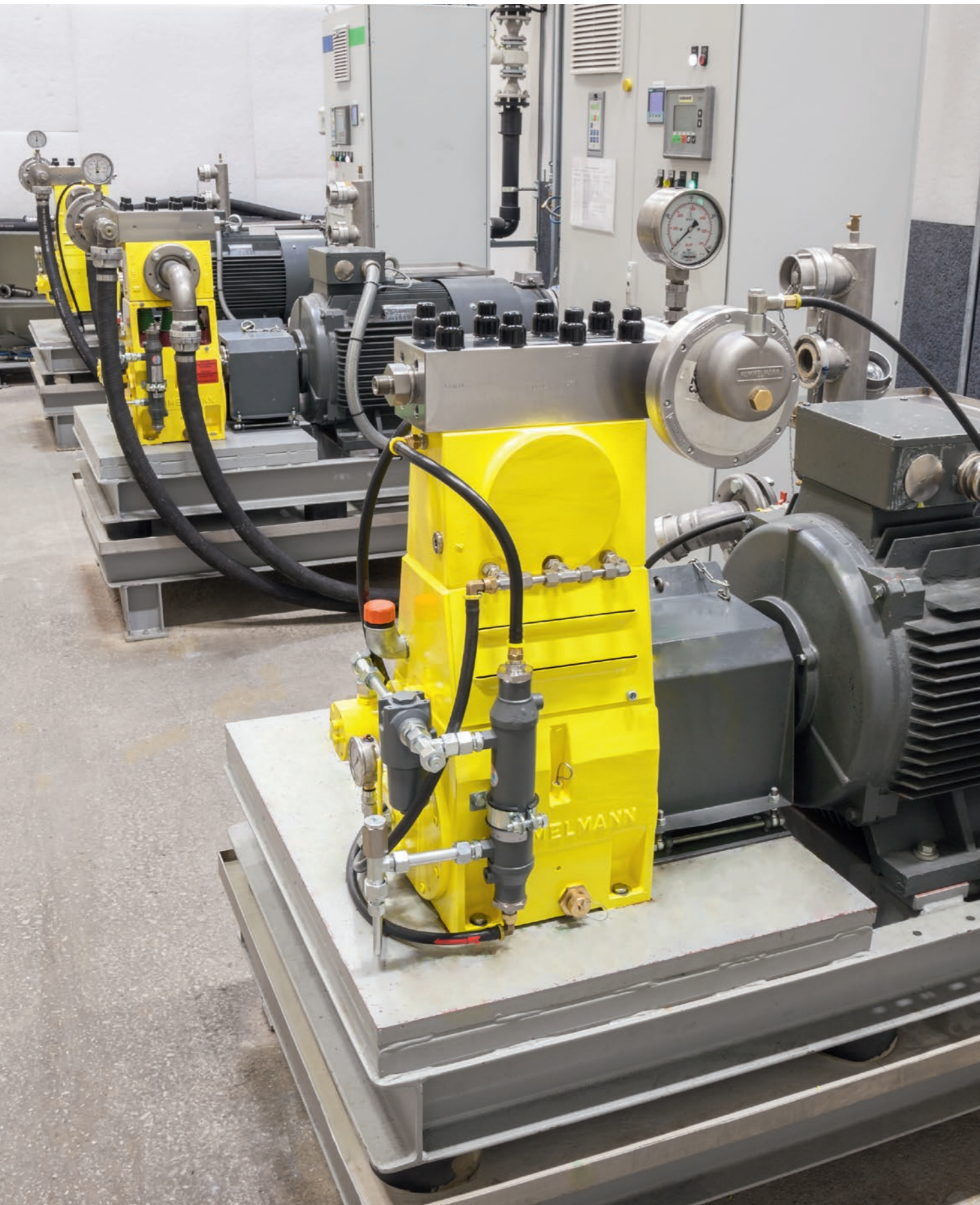
Test stations for all pump models, collation, evaluation and documentation of all relevant operating data.
